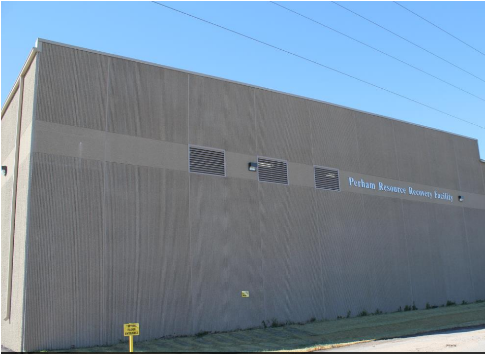
New Tipping Floor of the Perham Resource Recovery Facility
